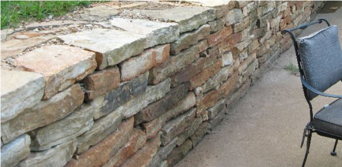
Above (option 1) Dry stacked sandstone (Photo credit: Gottschalk Sandstone Quarry)
