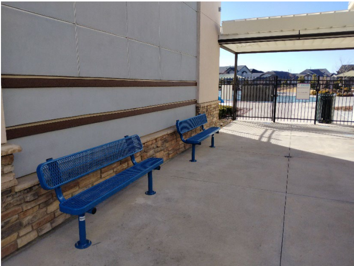
Figure 5- Bench additions at Pool Entry Gate
